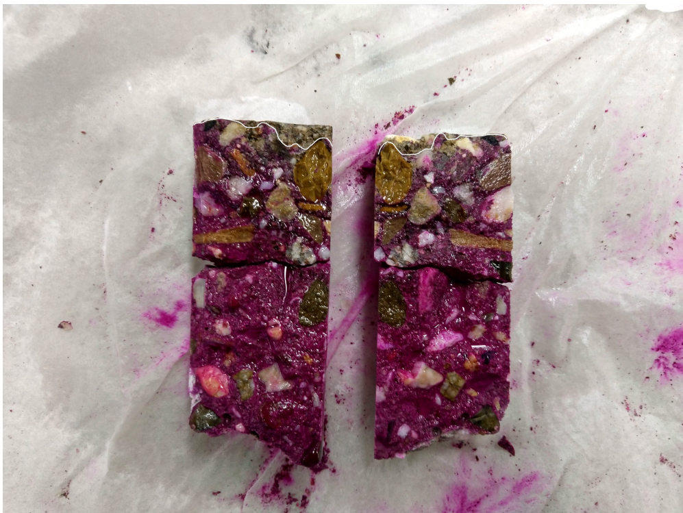
Figure E.42: Carbonation front C2-18.
