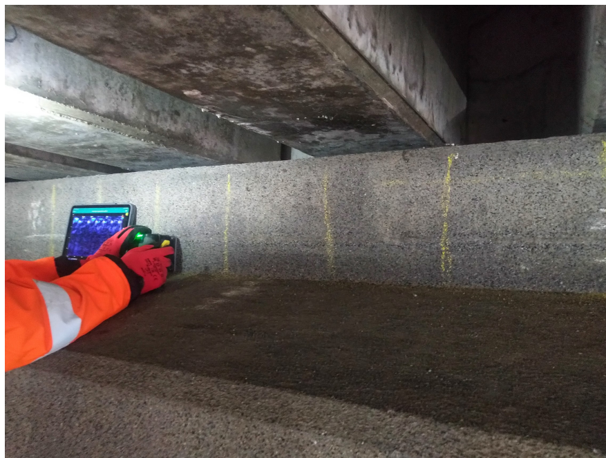
Figure 4.3: Using GPR to locate the reinforcement in the support beam.
