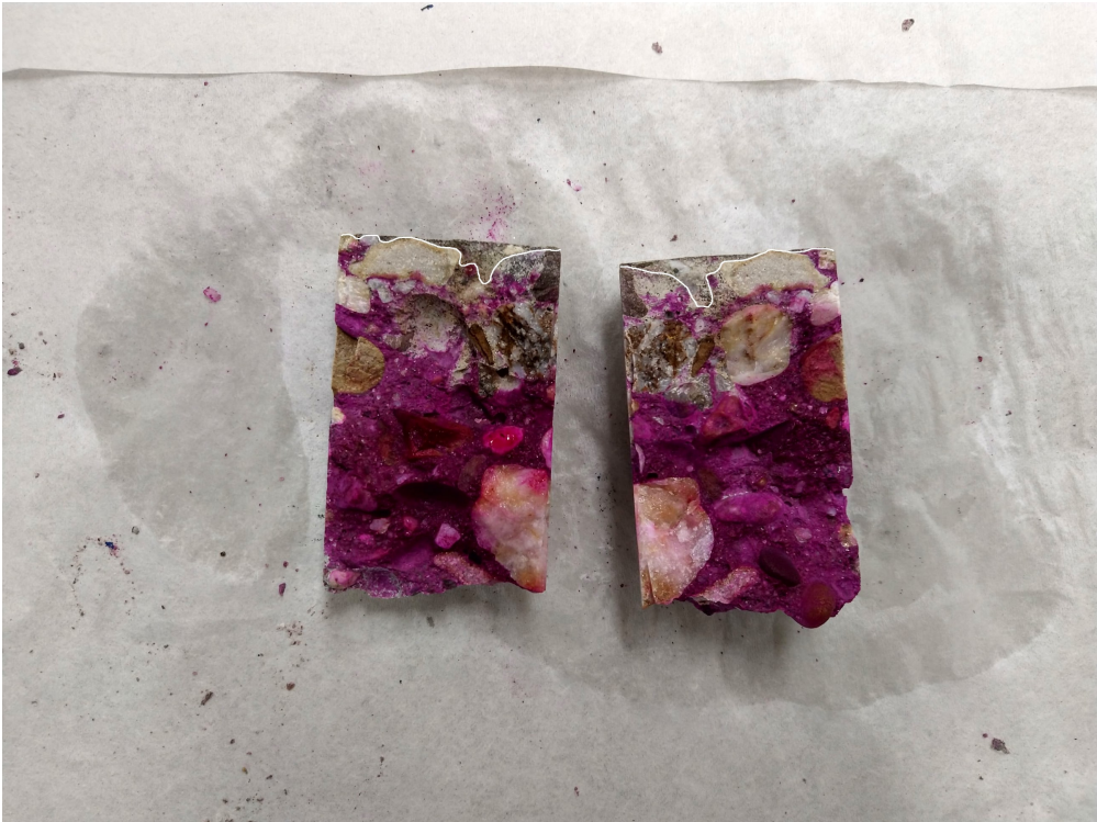
Figure E.40: Carbonation front C2-13.
