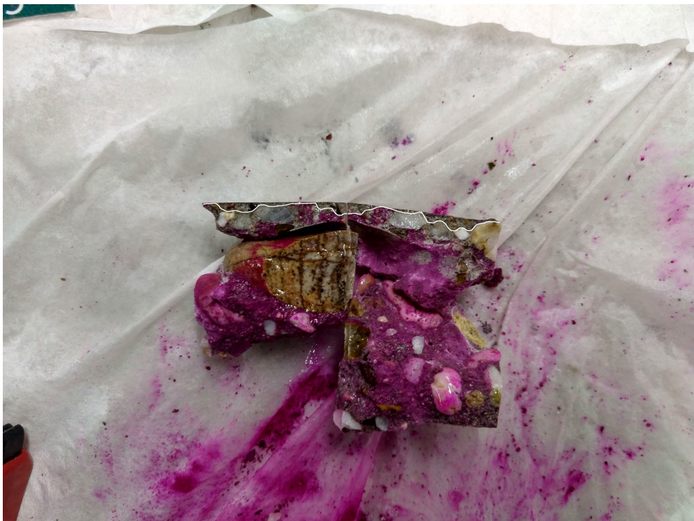
Figure E.38: Carbonation front C2-7.
