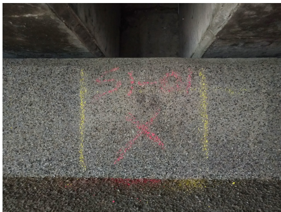
(a) Test location S1.
