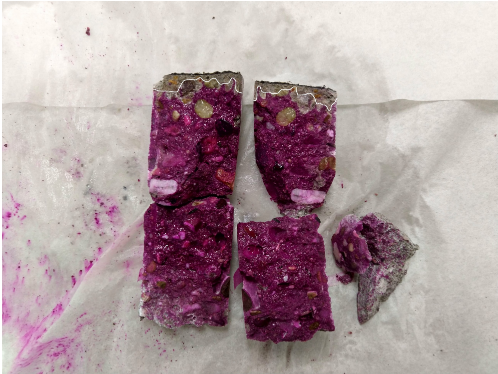
Figure E.33: Carbonation front C5.
