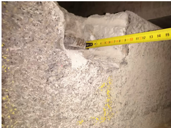
(a) Rebar location 1.
