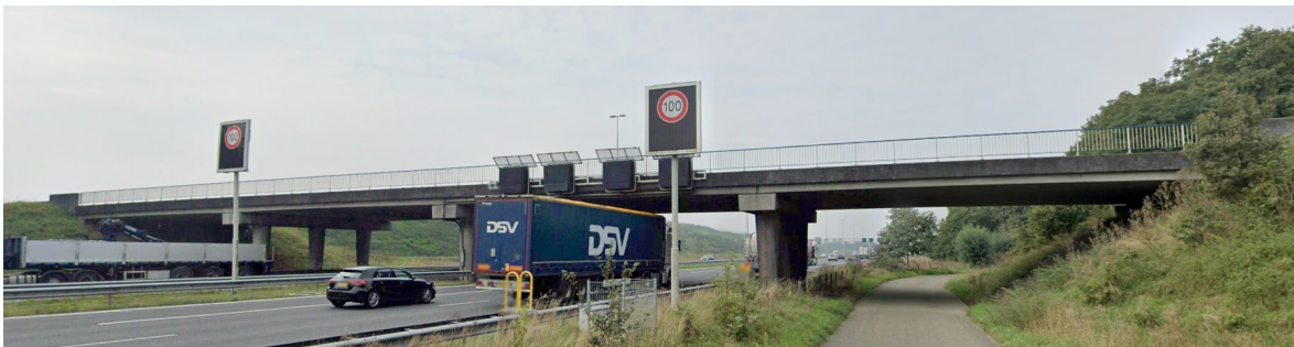
Figure 3.3: Sluinerweg viaduct as seen from the Blankenhuisweg.
