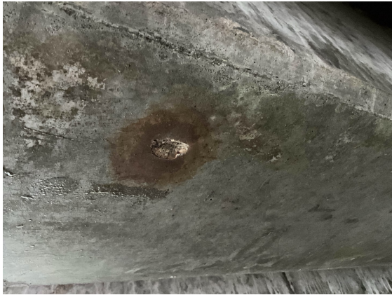
(e) Beam 14 bottom face.
