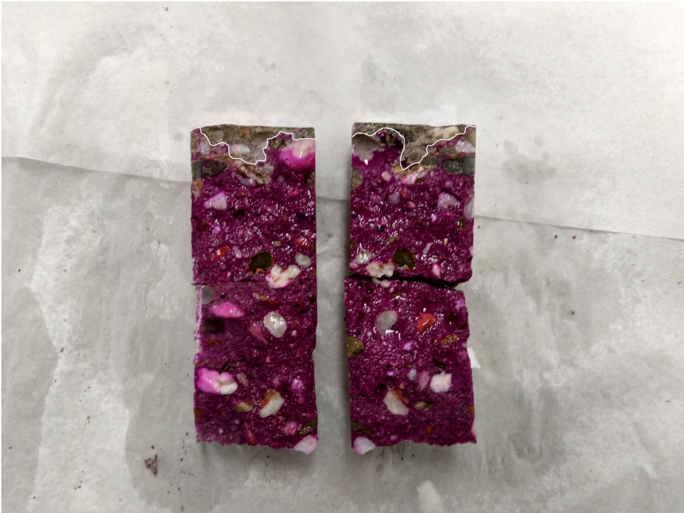
Figure E.39: Carbonation front C1-13.
