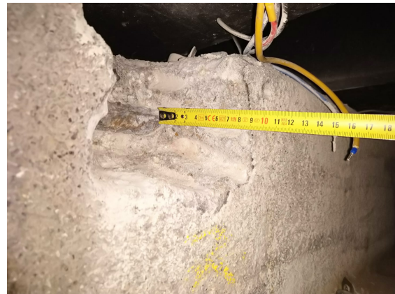
(b) Rebar location 2.
