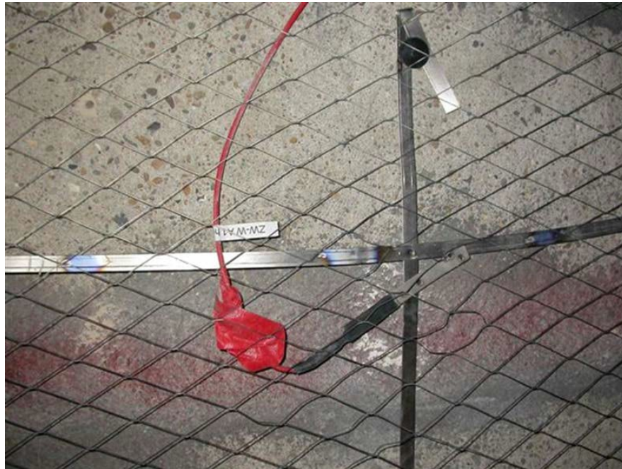
Figure 2.24: Connection between isolated copper cable, titanium mesh and plain titanium strip welded in-situ [81].
