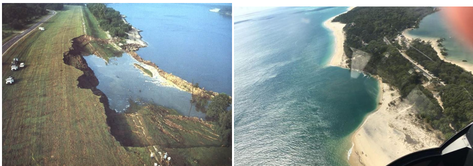
Figure 2.1: Damage to a river dike caused by a flow slide, from US Army Corps of Engineers ( left ) ( Rogers, 2012 ). A large collapse of beach at Inskip Point in Queensland due to a breaching event, from Rainbow Beach Helicopters Australia ( right ) ( BBC, 2018 ).
