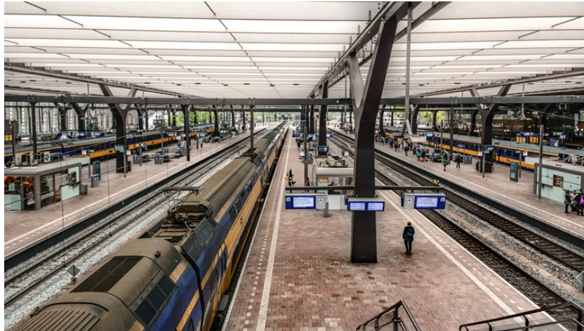
Figure 4.1: Interior of Rotterdam Central Station at railway track level. Image source: Rijnmond Public Broadcast (2020).
