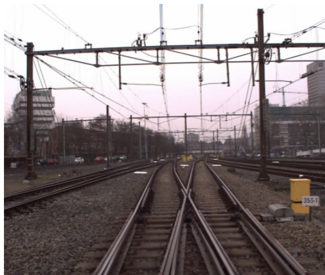
Figure 4.3: Sample image of the final study area at railway track level, captured by RILA system.
